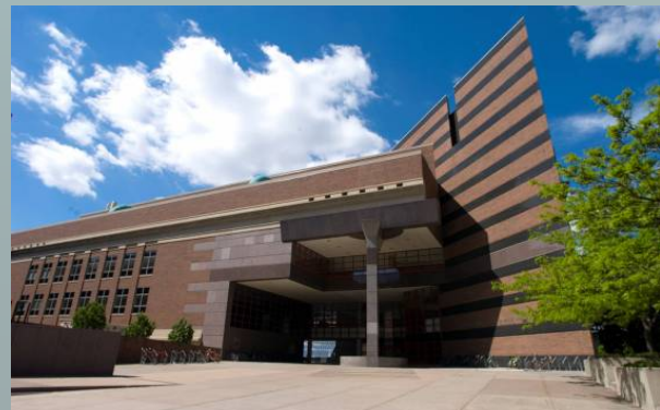
University of Minnesota Electrical Engineering/Computer Science Building
