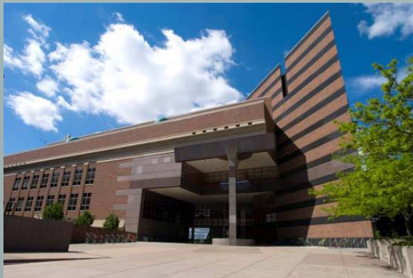
University of Minnesota Electrical Engineering/Computer Science Building
